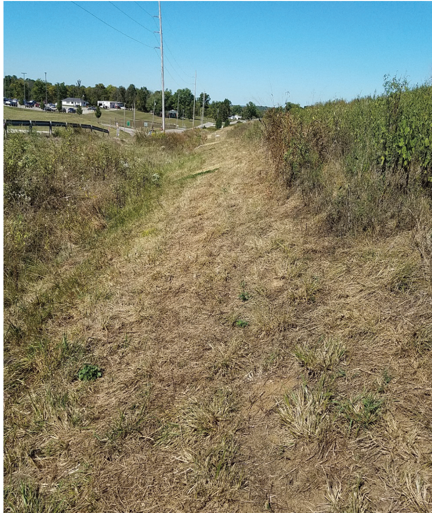
Photo 11: South of EV1 East Plant Cover System facing north
