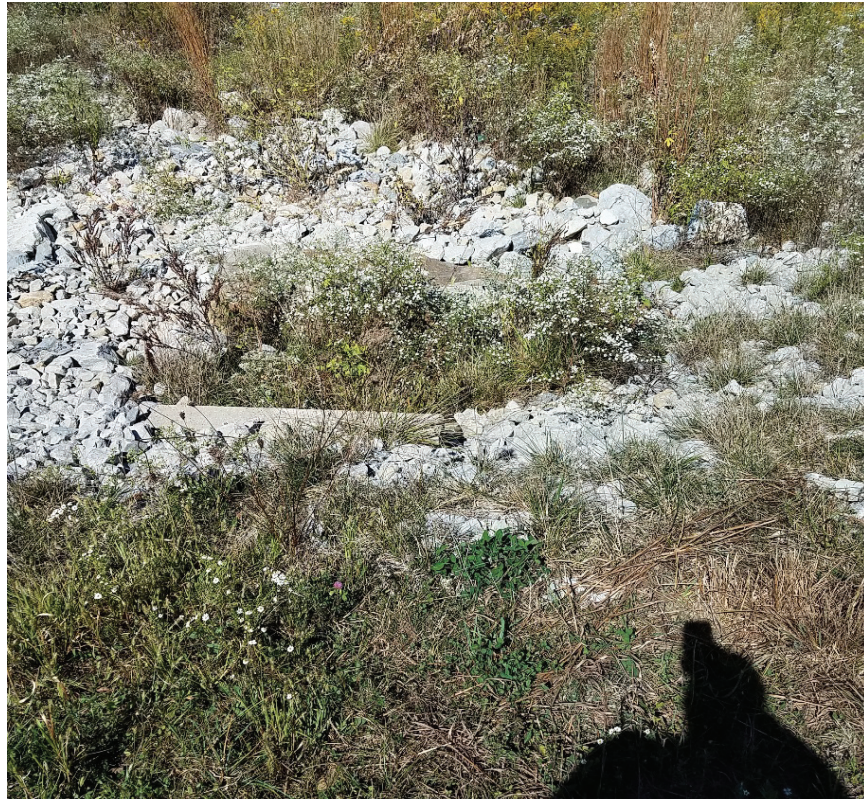
Photo 7: Drainage channel at ES6 East Plant Area Cover facing northeast.
