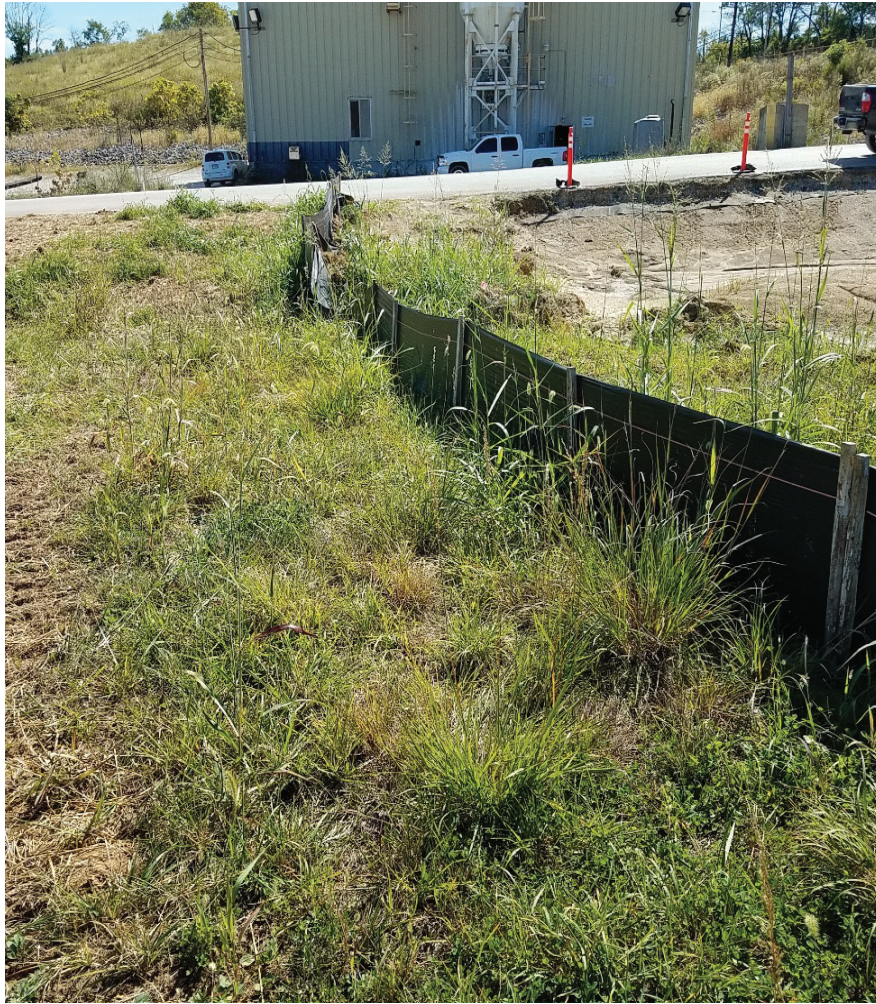
Photo 16: Facing east along EV7 East Plant Cover.
