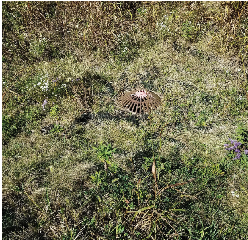
Photo 18: ES14 catch basin East Plant Area Cover.
