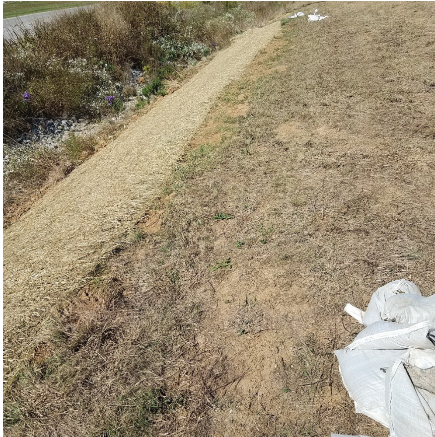
Photo 1: EV1 Vault Cover System west slope erosion area filled, seeded and straw placed.
