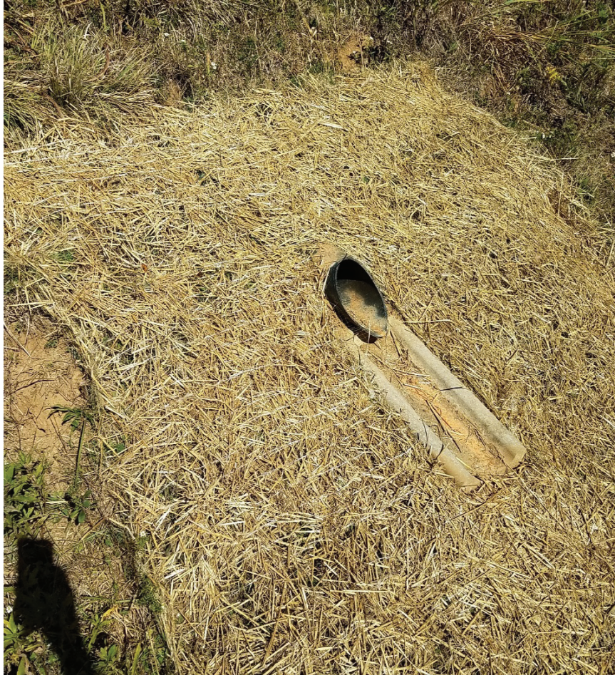
Photo 19: EV9 East Plant Area Cover erosion patch filled, seeded and straw placed.
