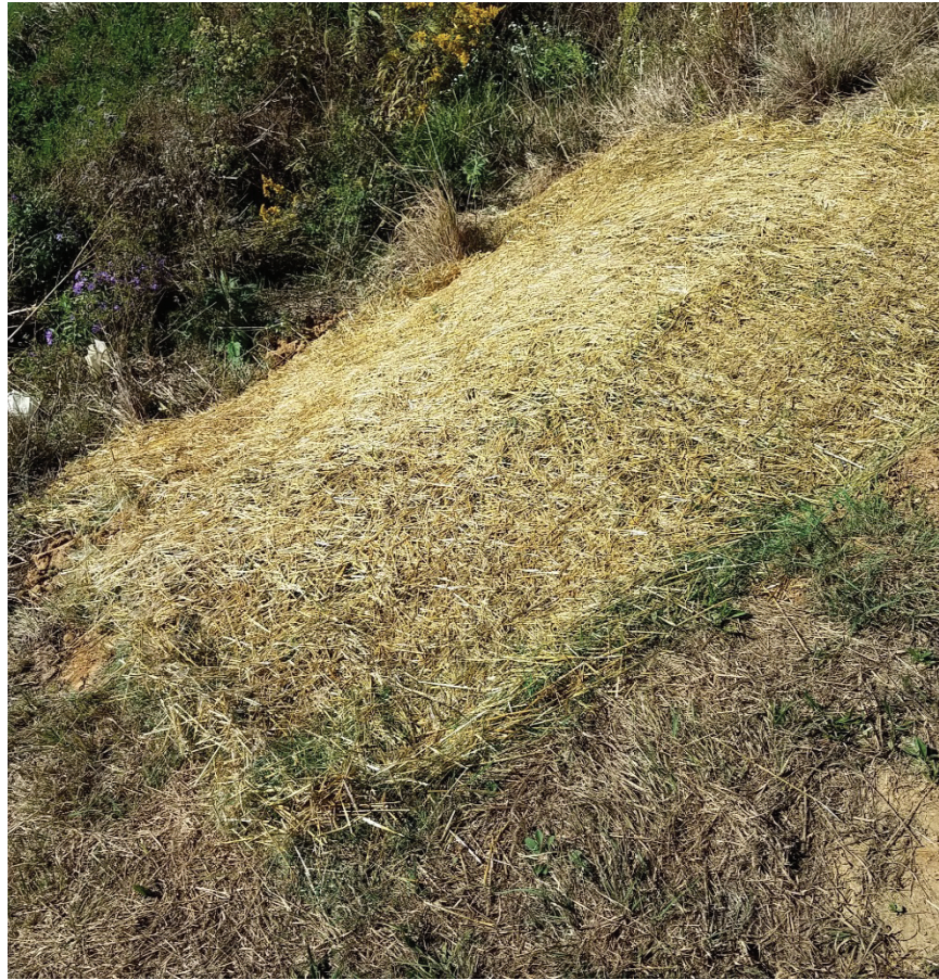
Photo 5: Erosion filled, seeded and straw placed at ES3.
