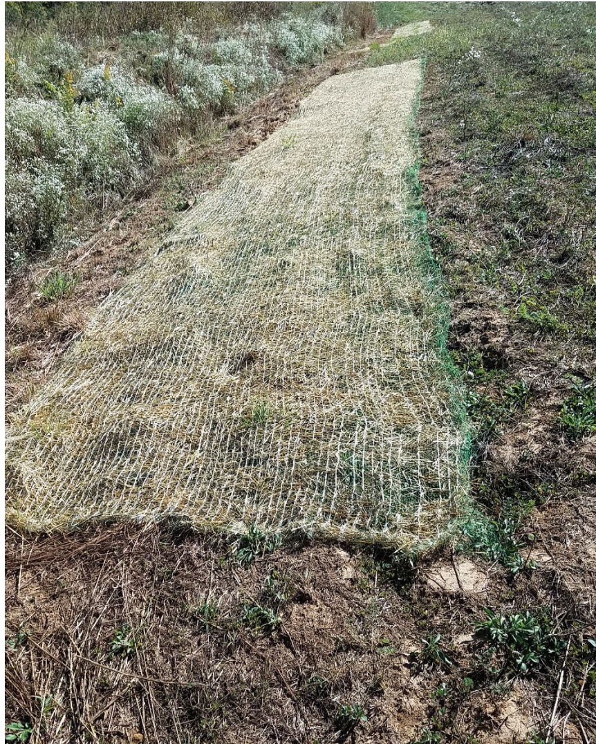
Photo 12: EV4 East Plant Area Cover vegetation filled, seeded and straw placed.
