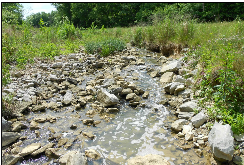
PHOTO 6: LOCATION 4 - LOOKING SOUTHEAST (UPSTREAM).
