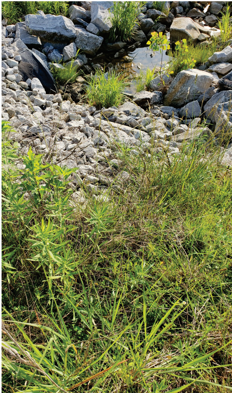
Photo 7: Drainage at ES6 facing east at EV5
