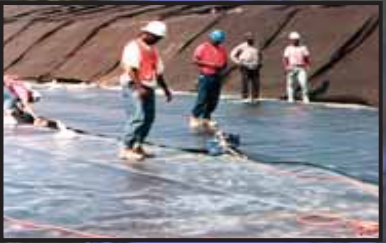
High Density Polyethylene (HDPE) Liner Seaming
