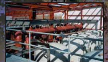
INSTALLED GRANULAR ACTIVATED CARBON VESSELS
