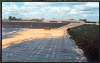
Placement of Drainage Layer over HDPE Liner
