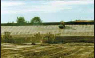
Placement of Clay Layer of Vault Cap
