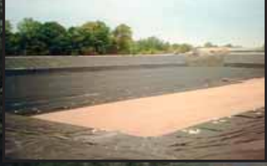
High Density Polyethylene (HDPE) Liner Placement
