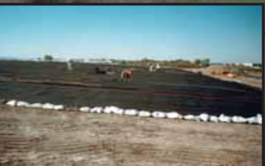
Placement of HDPE Liner as Part of Vault Cap
