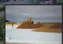
PLACEMENT OF DRAINAGE LAYER OVER GCL
