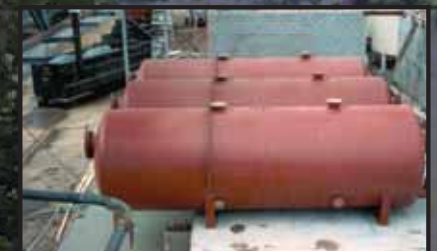
SAND FILTER INSTALLATION
