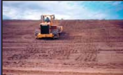
Placement of Clay Layer of Vault Cap
