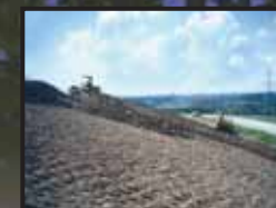
PLACEMENT OF GRADING FILL
