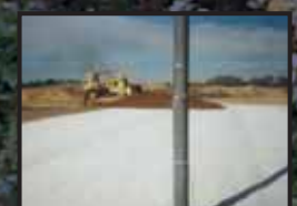
PLACEMENT OF DRAINAGE LAYER OVER GCL
