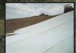
PLACEMENT OF DRAINAGE LAYER OVER GCL
