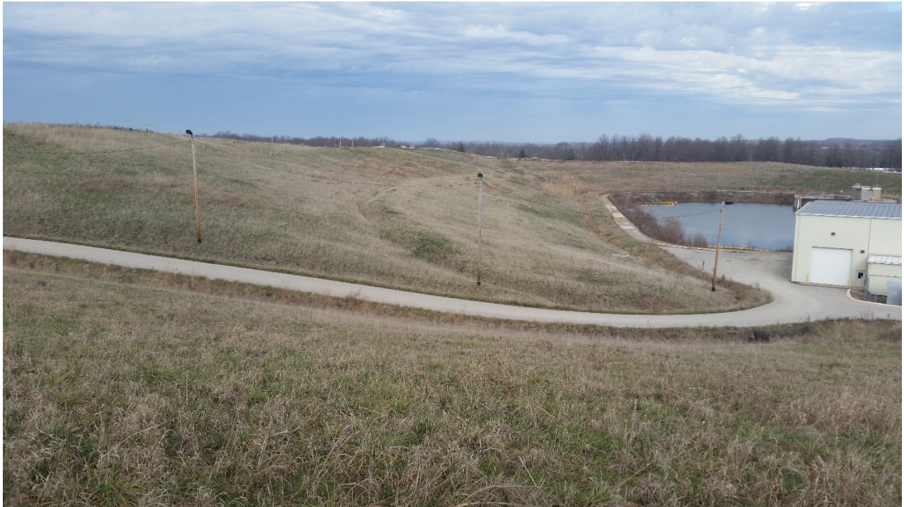
Photo 20: ES1 and ES2 drainage swale facing north.
