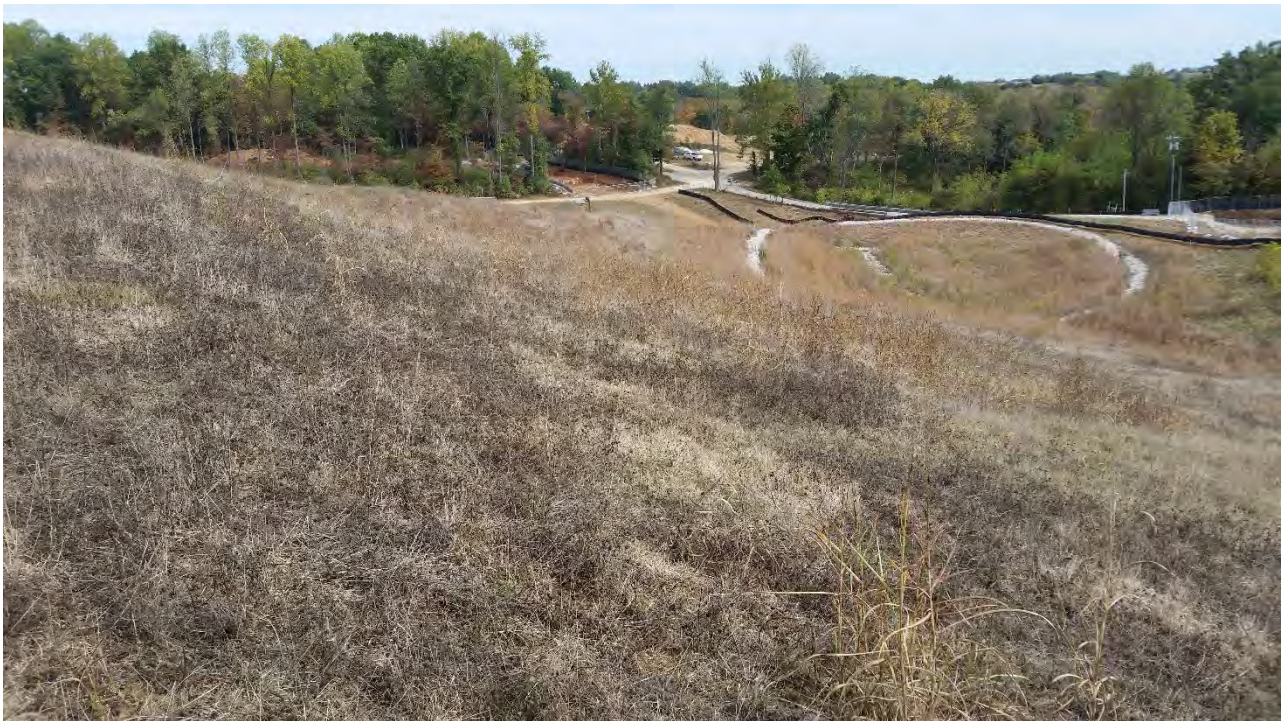
Photo 5: EV4 East Plant Area cover facing northeast
