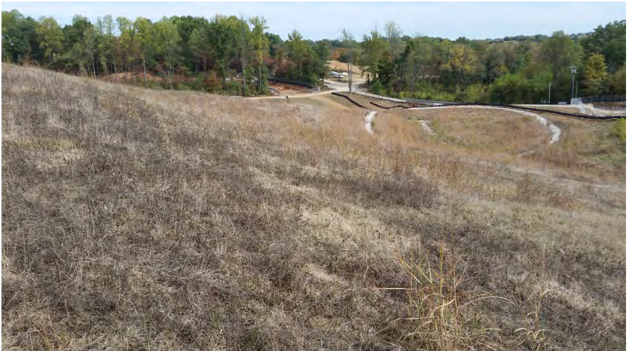
Photo 27: ES11 detention basin #5 facing north
