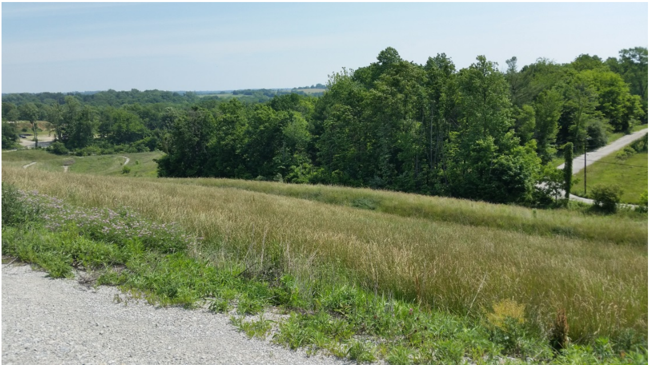
Photo 7: EV5 East Plant Area cover facing northeast
