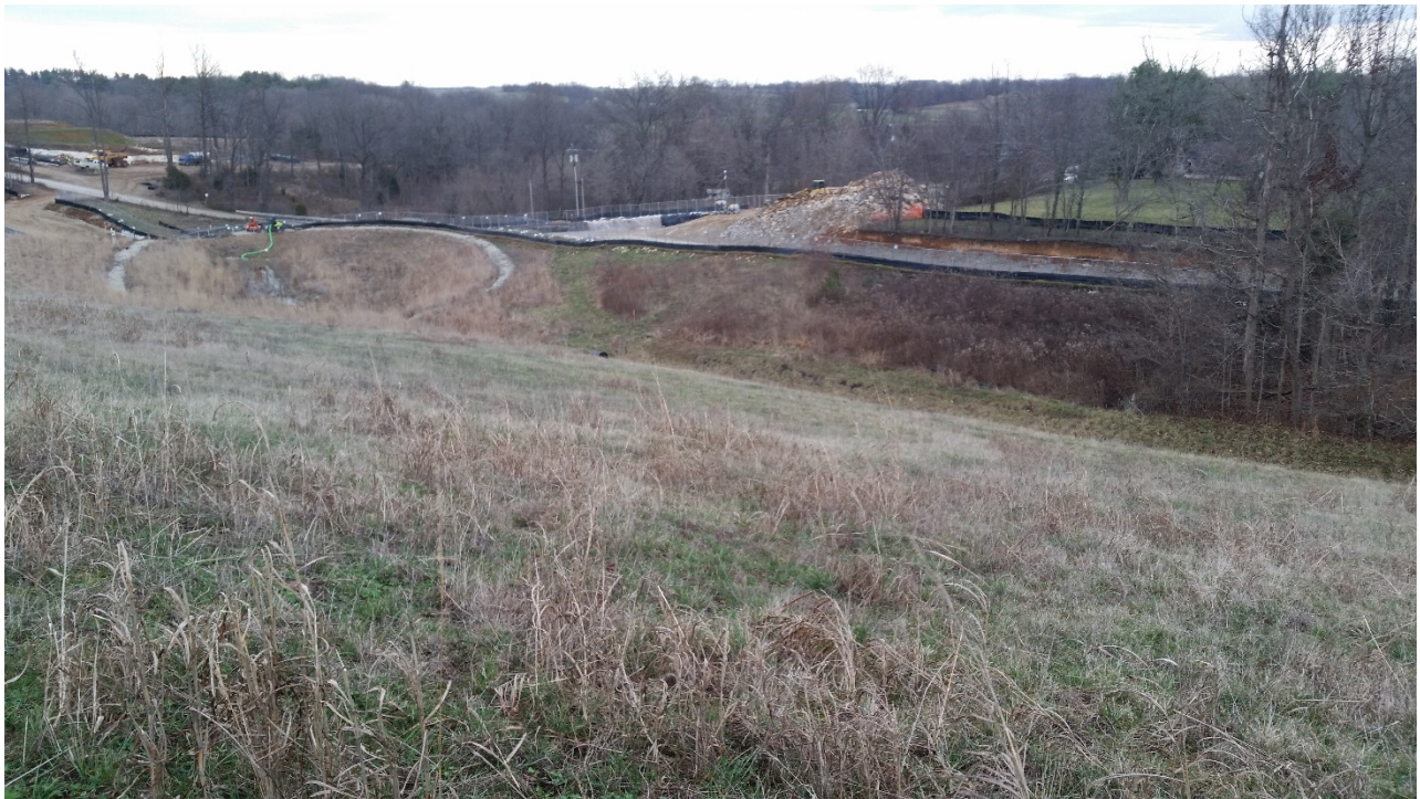
Photo 8: EV5 East Plant Area cover facing northeast.
