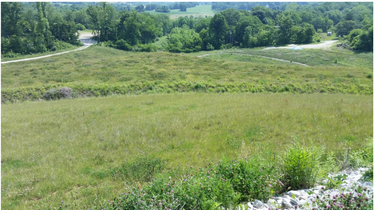
Photo 6: EV4 East Plant Area cover facing northeast
