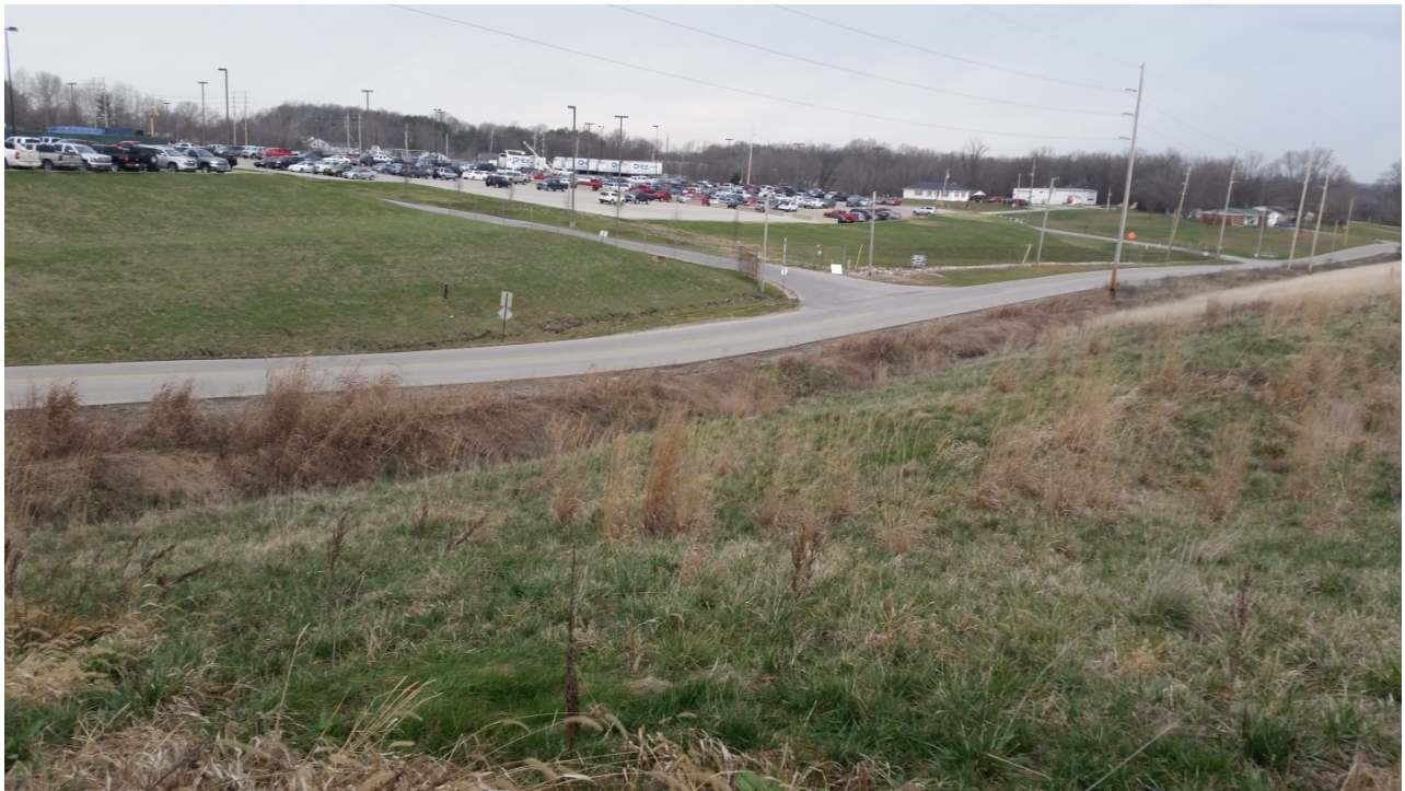
Photo 1: EV1 Vault cover facing northwest.
