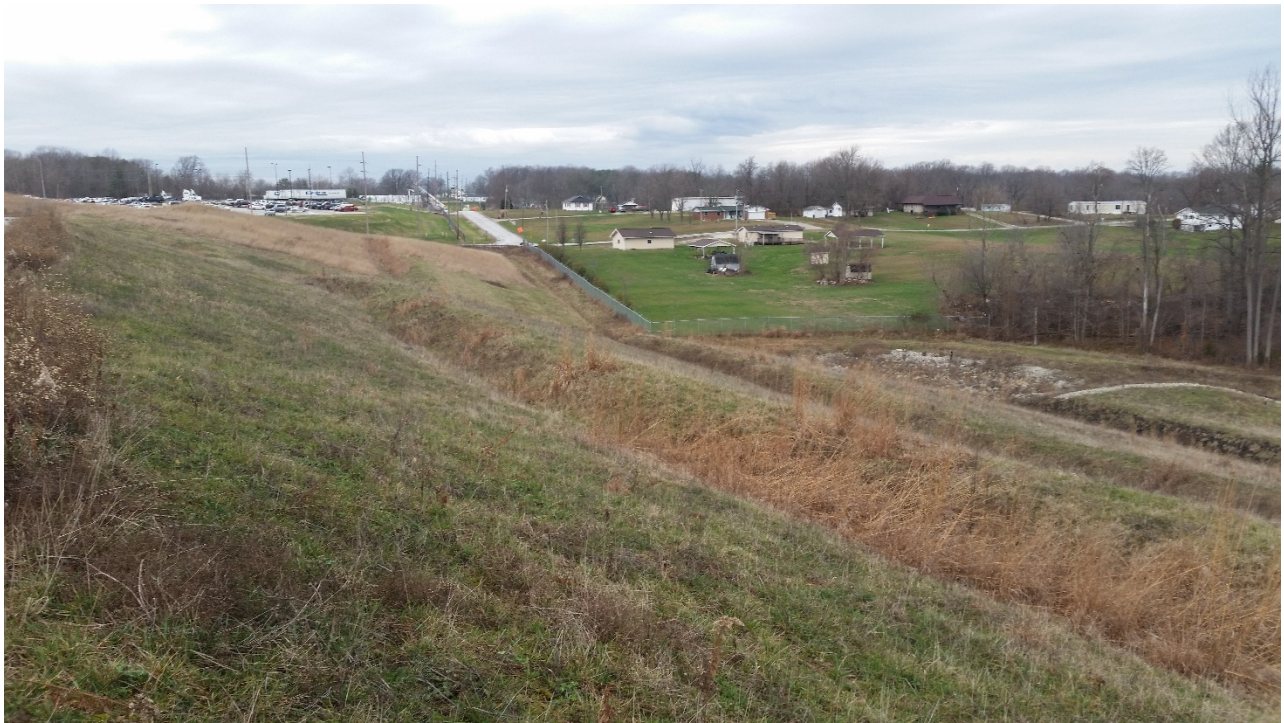
Photo 22: ES4 drainage swale facing west.
