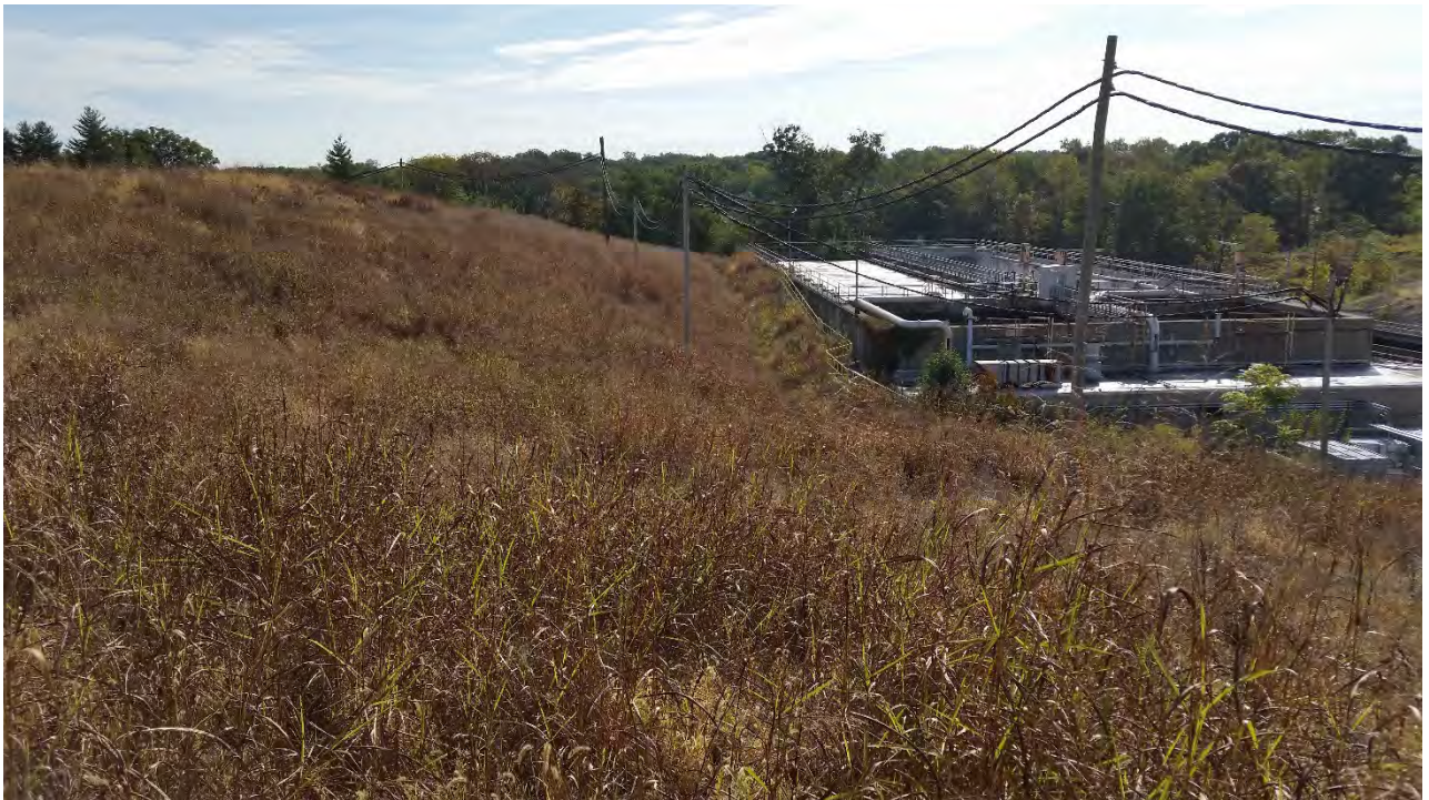
Photo 11: EV6 East Plant Area cover facing southwest
