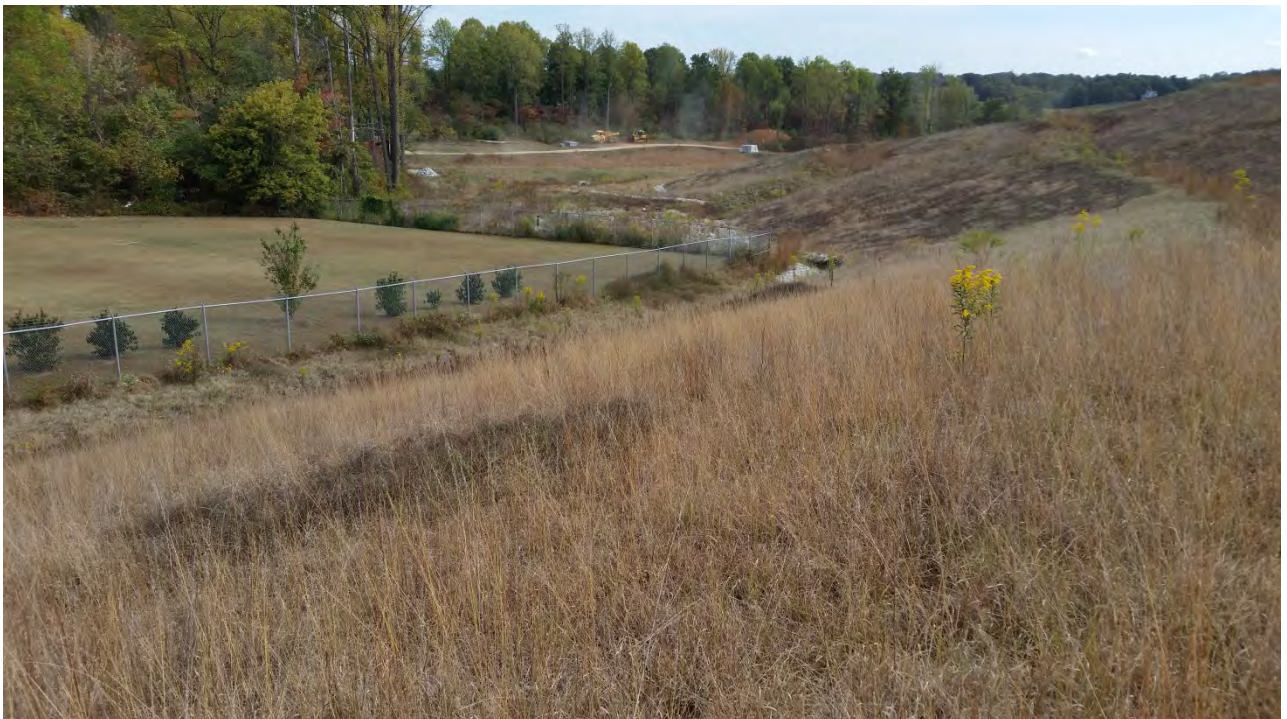
Photo 22: ES5 drainage swale facing northeast
