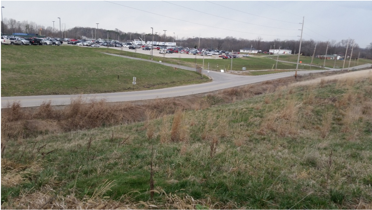
Photo 36: WV1 West Plant Area cover facing northwest.
