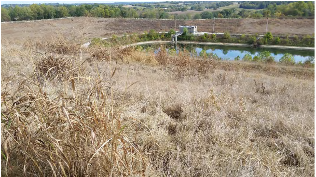
Photo 19: ES2 drainage swale facing north
