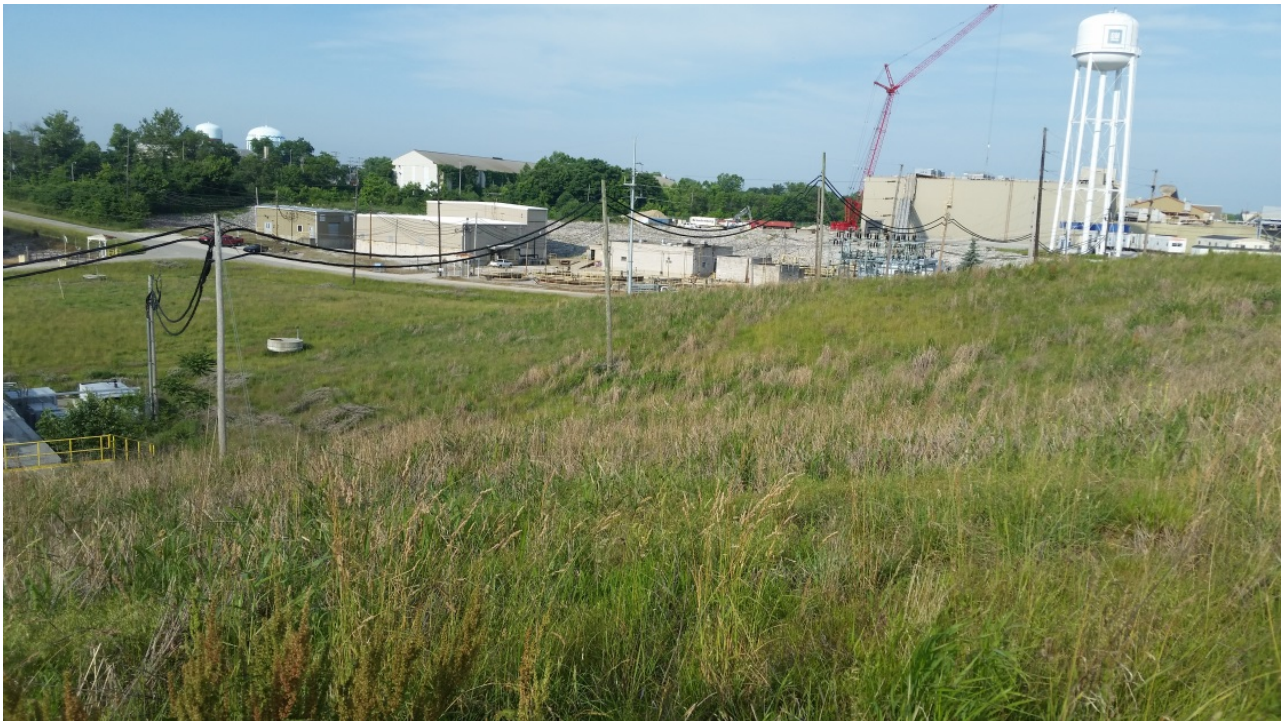
Photo 10: EV6 East Plant Area cover facing southwest
