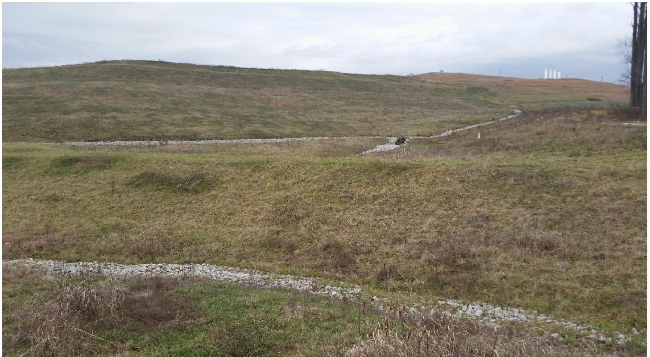
Photo 7: EV4 East Plant Area cover facing southwest.
