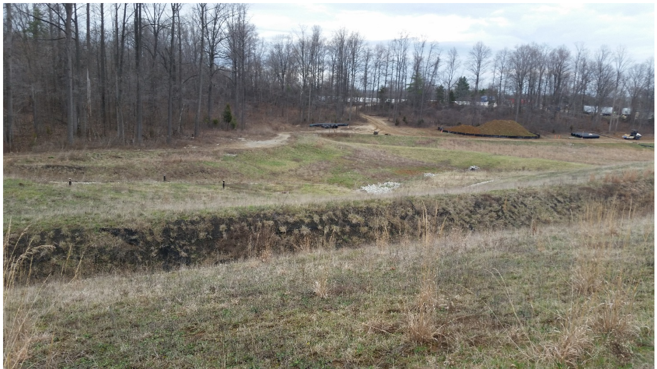
Photo 25: ES6 facing northeast.
