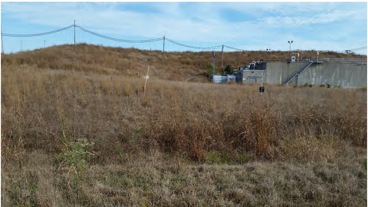
Photo 12: EV7 East Plant Area cover facing north
