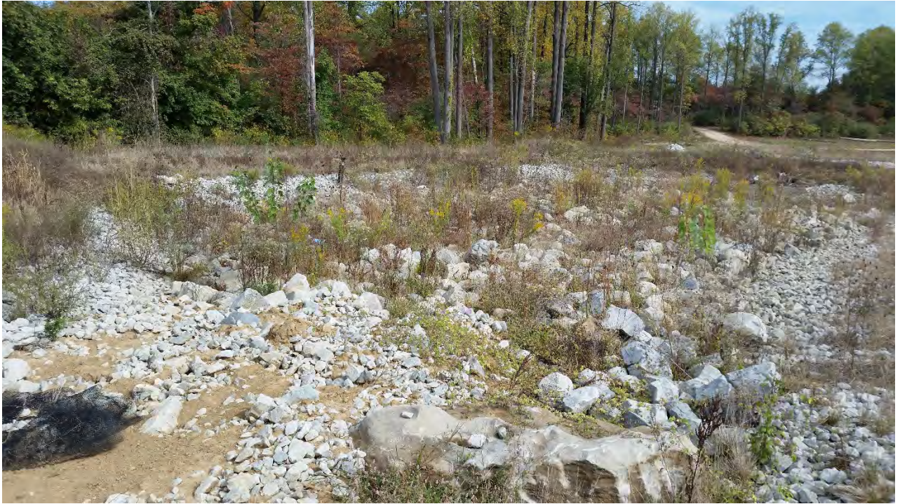
Photo 26: ES9 rip rap erosion at storm drain into detention basin #2 facing west
