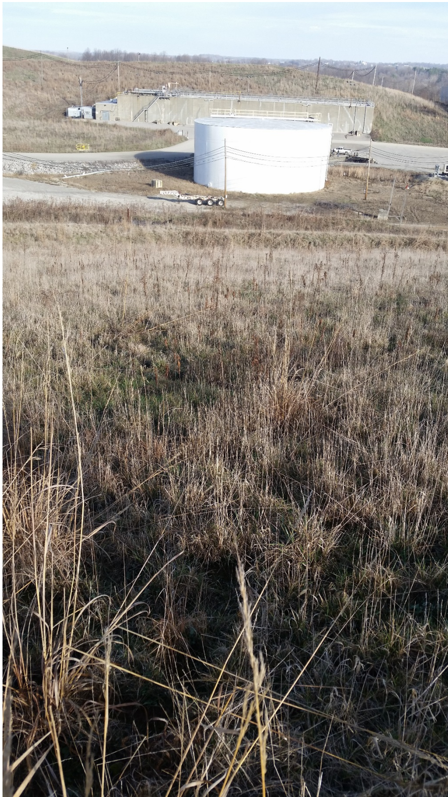
Photo 18: EV9 East Plant Area cover facing north.
