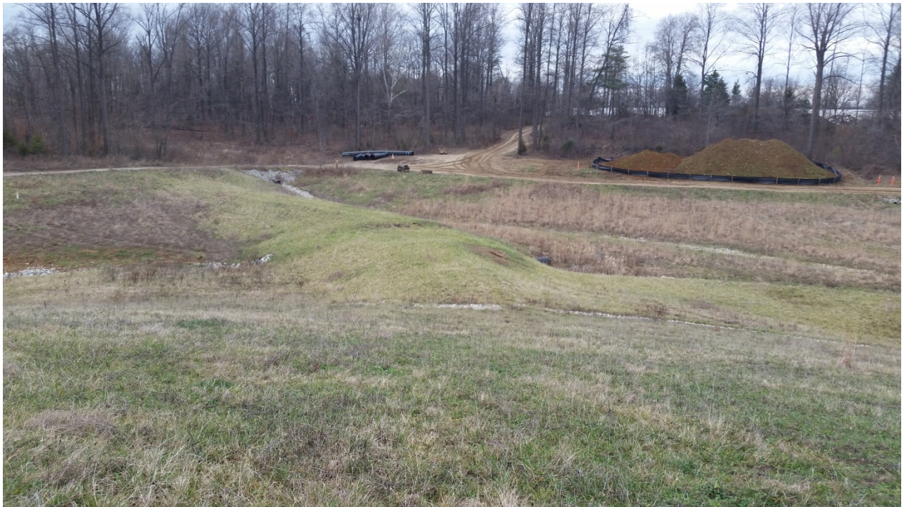
Photo 5: EV3 East Plant Area cover facing north.
