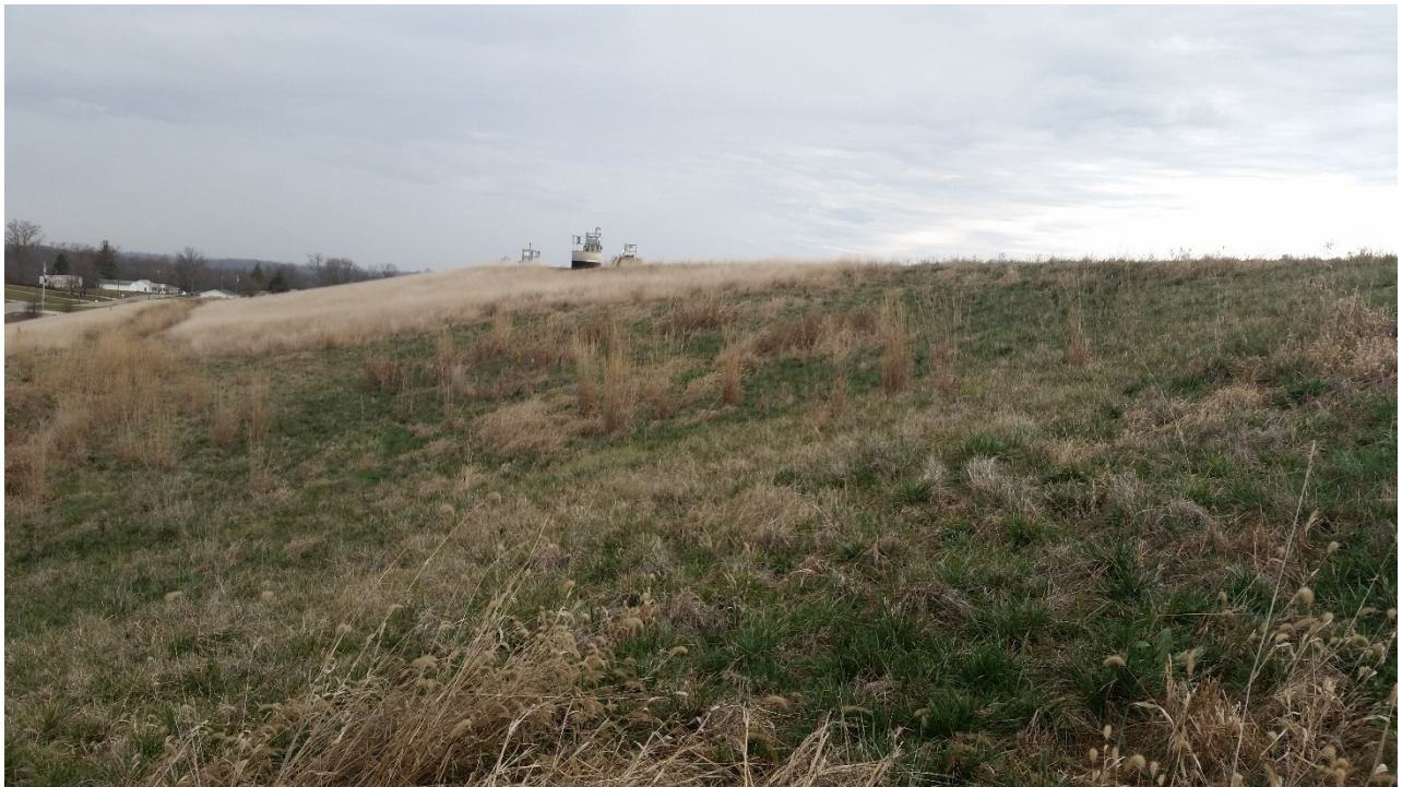
Photo 2: EV1 Vault cover facing North.
