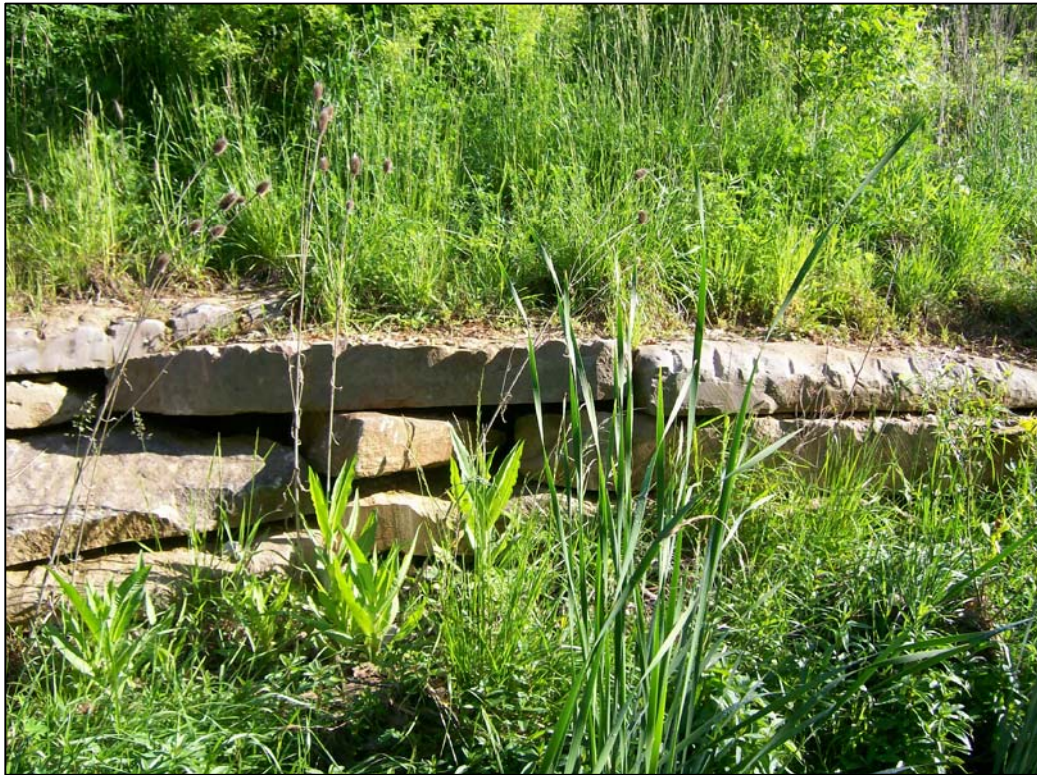
FIGURE 6.2 - PARCEL 6, LOCATION 6, LOOKING NORTH BANK
