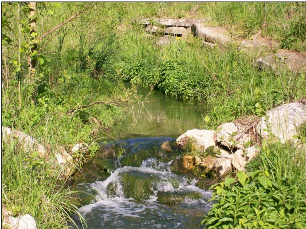
FIGURE 7.2 - PARCEL 5, LOCATION 7, ROCK CURRENT DEFLECTOR
