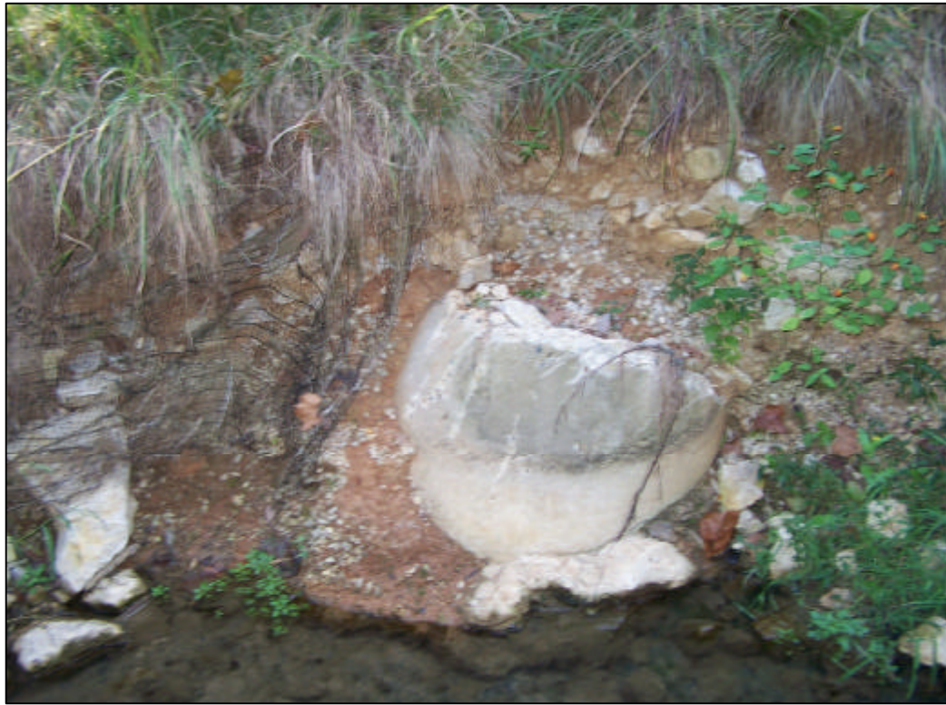
FIGURE 17.4 - PARCEL 11, LOCATION 17, EAST BANK
