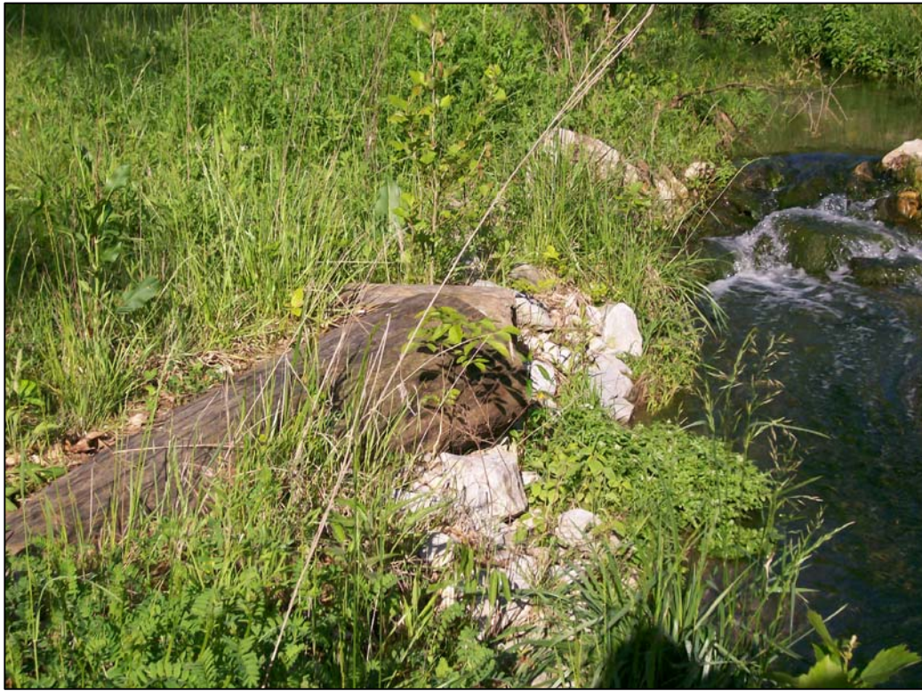
FIGURE 7.3 - PARCEL 5, LOCATION 7, LOG DEFLECTOR ON SOUTH BANK
