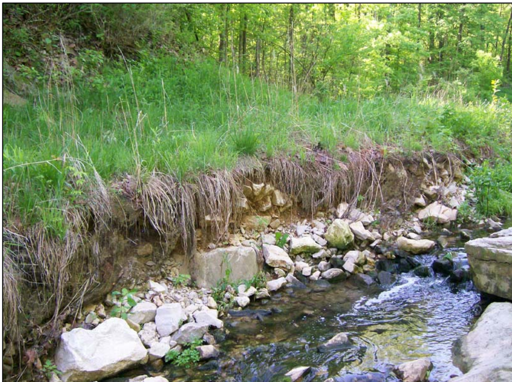
FIGURE 20.2 - PARCEL 11, LOCATION 20, LOOKING EAST BANK
