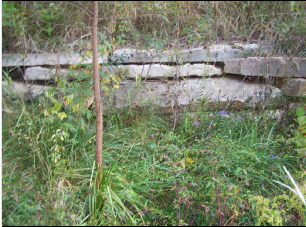
FIGURE 5.3 - PARCEL 5, LOCATION 5, LOOKING NORTHWEST (BANK STABILIZATION)
