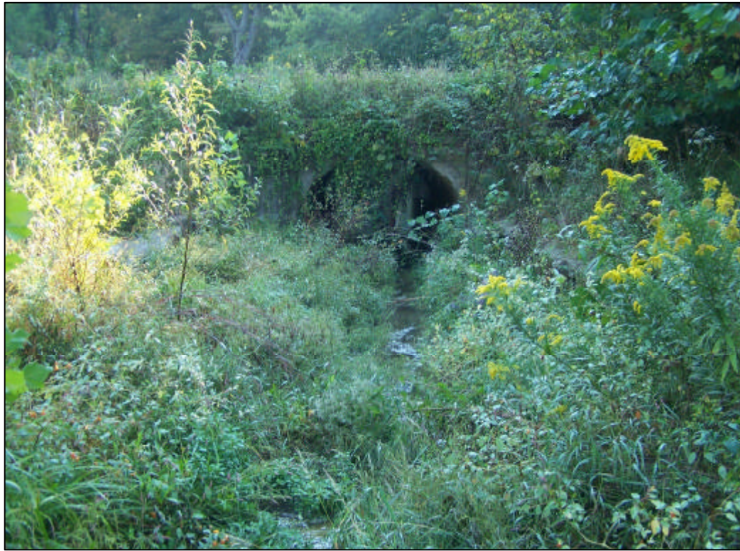
FIGURE 6.1 - PARCEL 5, LOCATION 6, LOOKING DOWNSTREAM (NORTHEAST)
