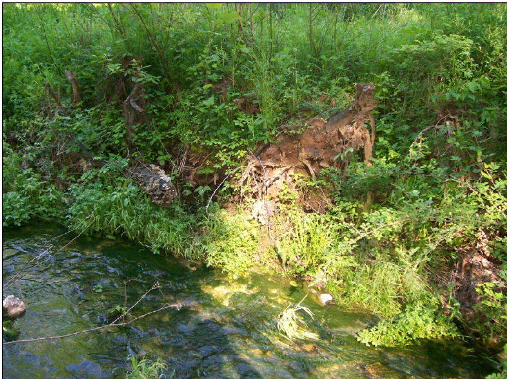
FIGURE 16.4 - PARCEL 8, LOCATION 16, SPECIAL LOOKING WEST/ ROOT WAD FEATURE
