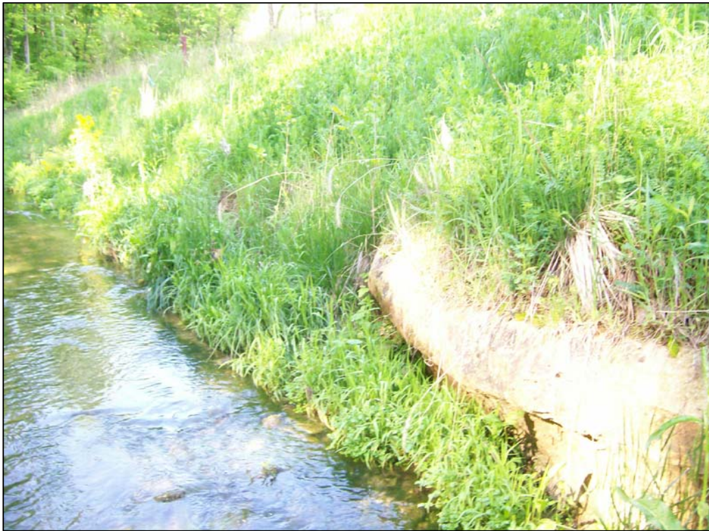
FIGURE 15.3 - PARCEL 8, LOCATION 15, LOOKING WEST BANK
