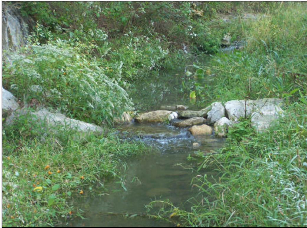
FIGURE 12.5 - PARCEL 10, LOCATION 12, LOOKING AT ROCK CURRENT DEFLECTOR (SOUTHWEST)
