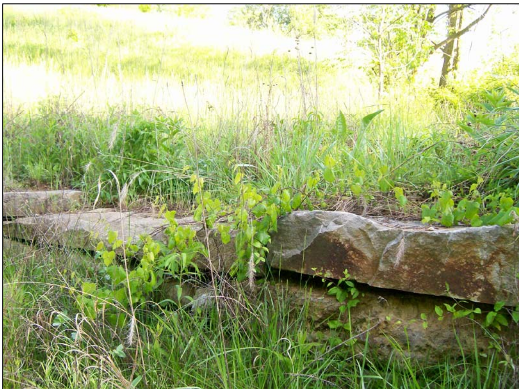
FIGURE 9.3 - PARCEL 5, LOCATION 9, LOOKING NORTH BANK
