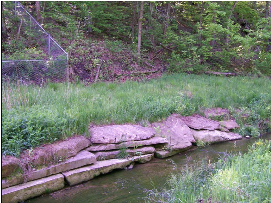
FIGURE 22.2 - PARCEL 11, LOCATION 22, LOOKING EAST BANK
