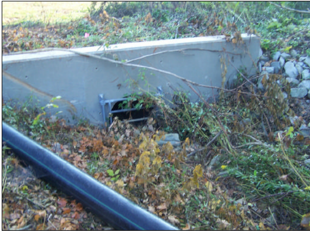
FIGURE 1.4 - PARCEL 3, LOCATION 1, CULVERT INLET
