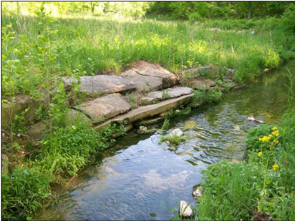
FIGURE 16.5 - PARCEL 8, LOCATION 16, SPECIAL LOOKING NORTHWEST/ ROUGHBACK BANK STABILIZATION
