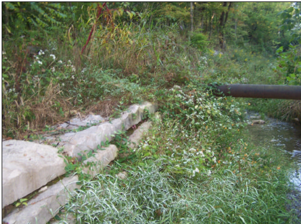
FIGURE 10.2 - PARCEL 7, LOCATION 10, LOOKING EAST BANK
