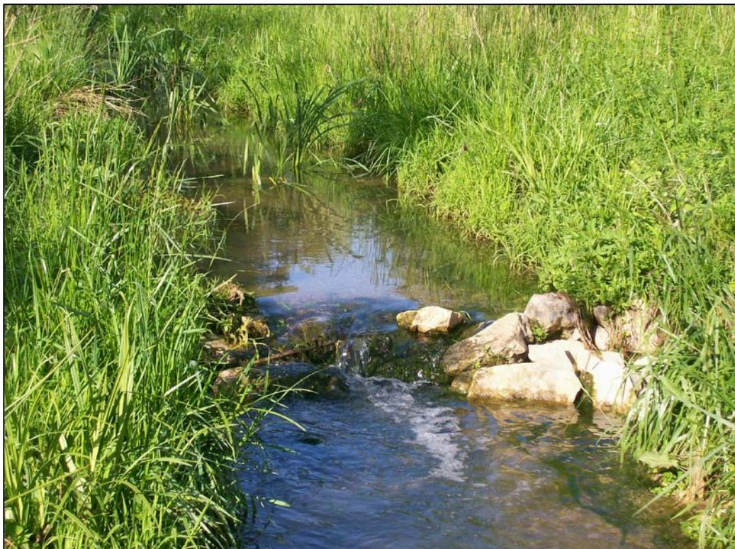
FIGURE 6.3 - PARCEL 6, LOCATION 6, ROCK CURRENT DEFLECTOR (SOUTHWEST)
