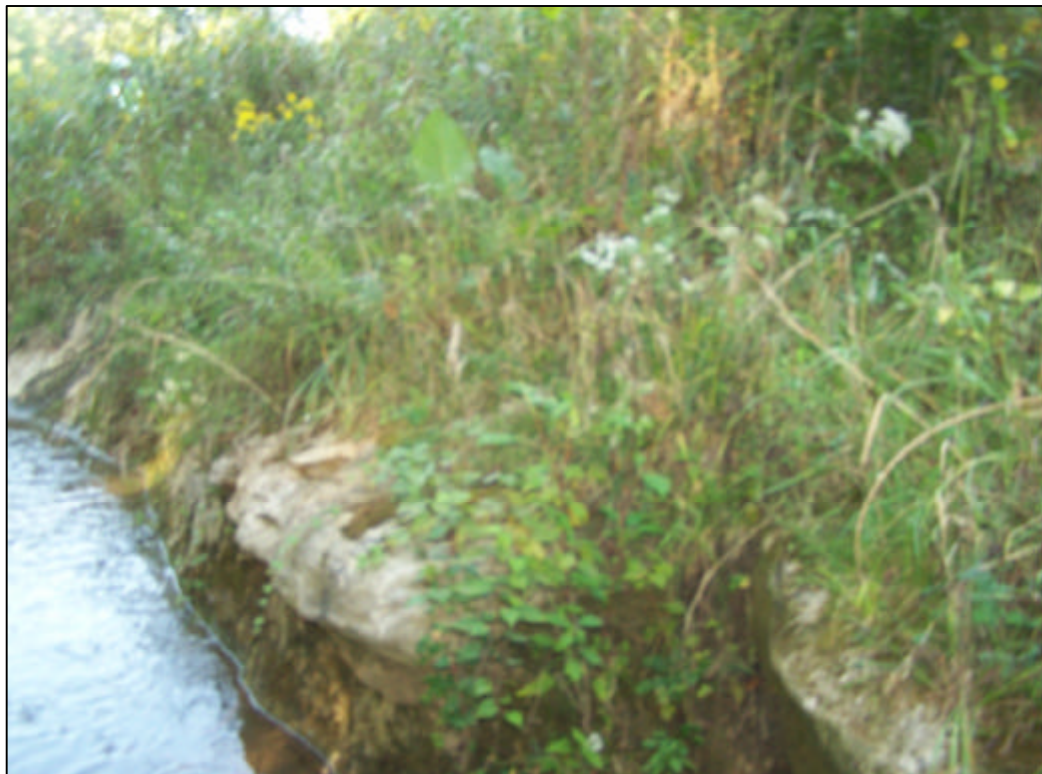
FIGURE 11.3 - PARCEL 9, LOCATION 11, LOOKING WEST BANK
