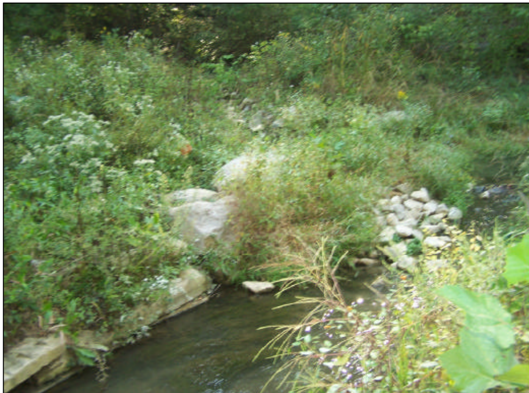
FIGURE 16.0 - PARCEL 8, LOCATION 16, LOOKING TRIBUTARY (EAST)
