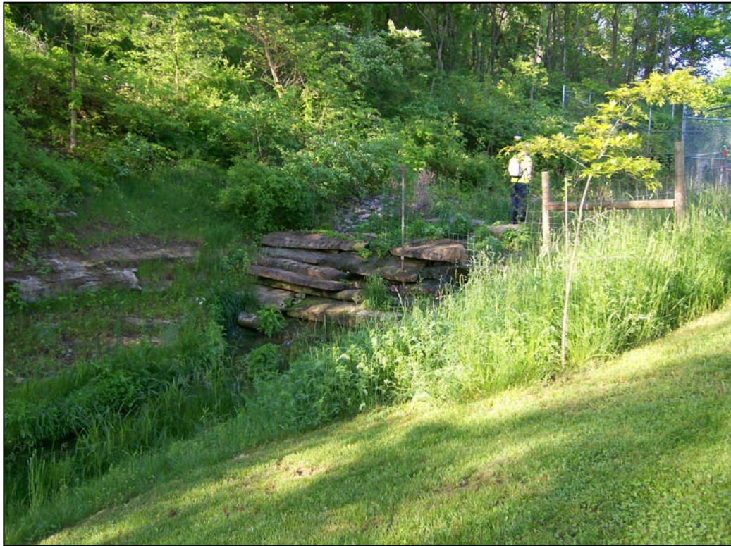
FIGURE 4.4 - PARCEL 205, LOCATION 4, OUTFALL SPECIAL LOOKING SOUTHWEST
