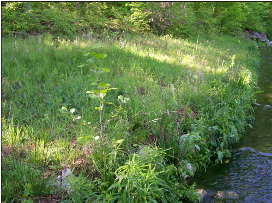
FIGURE 15.2 - PARCEL 8, LOCATION 15, LOOKING EAST BANK
