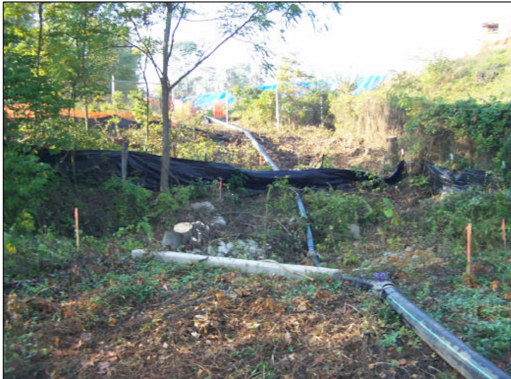
FIGURE 1.3 - PARCEL 3, LOCATION 1, LOOKING SOUTH
