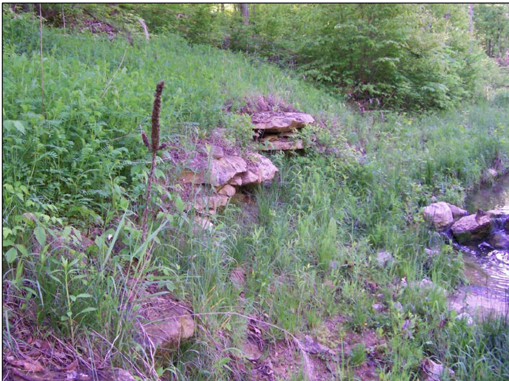
FIGURE 17.2 - PARCEL 8, LOCATION 17, LOOKING EAST BANK
