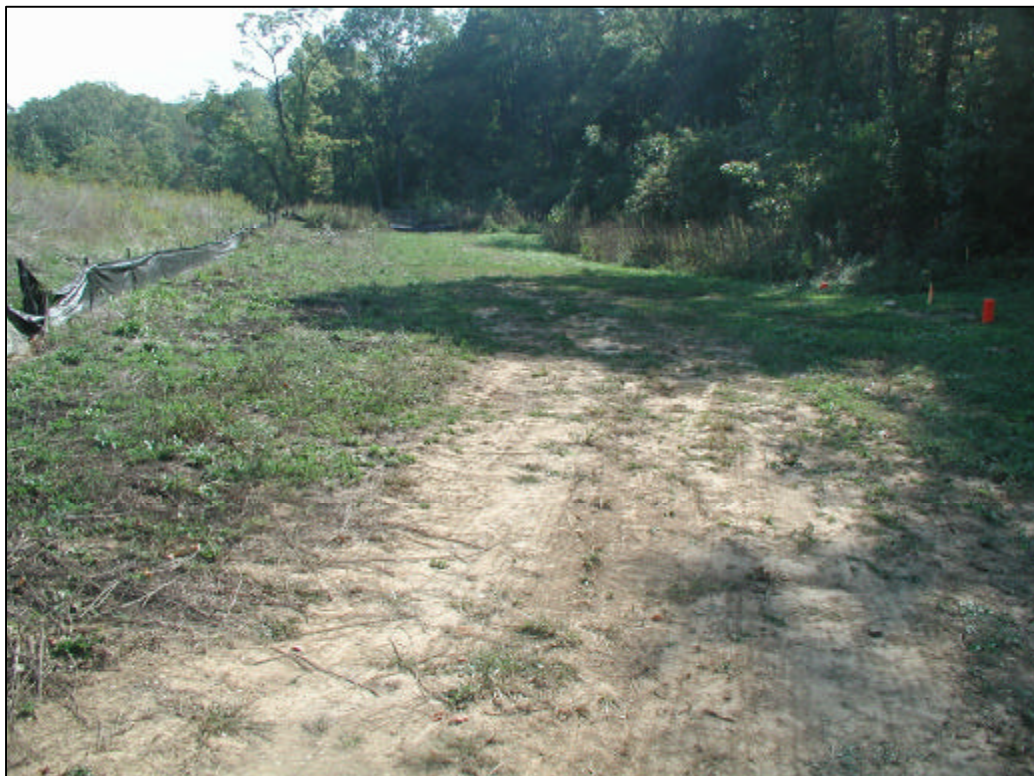
FIGURE 58 - CLEARED VEGETATION, PARCEL 205, 9/23/2008
