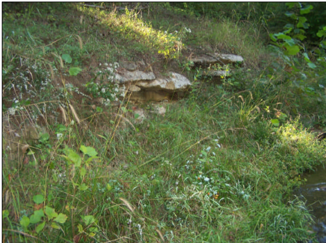
FIGURE 14.2 - PARCEL8, LOCATION 14, LOOKING EAST BANK
