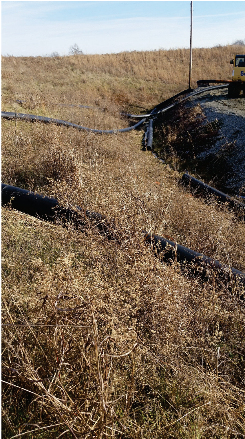
Photo 9: Temporary pumping lines in ES1 East Plant Area Cover at north end of Pond
