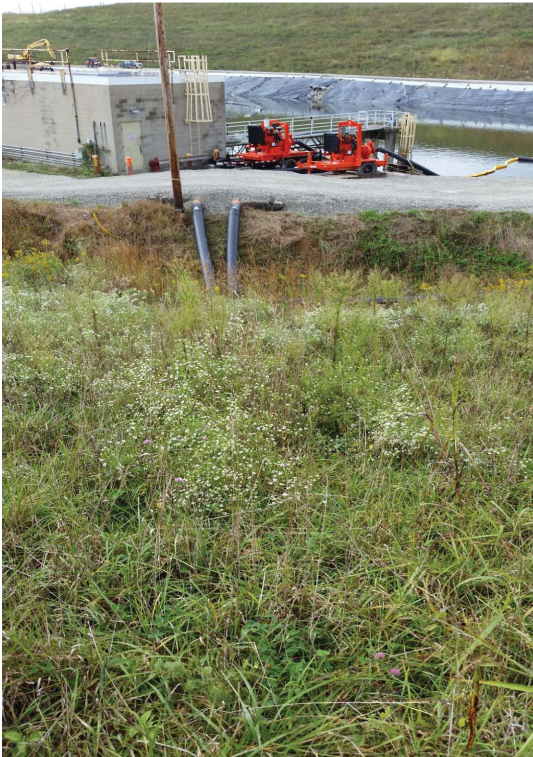
Photo 11: Vegetative growth along EV5 East Plant Area facing west towards lagoon
