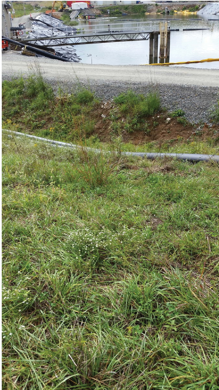
Photo 10: Looking south towards Stormwater Pond.
