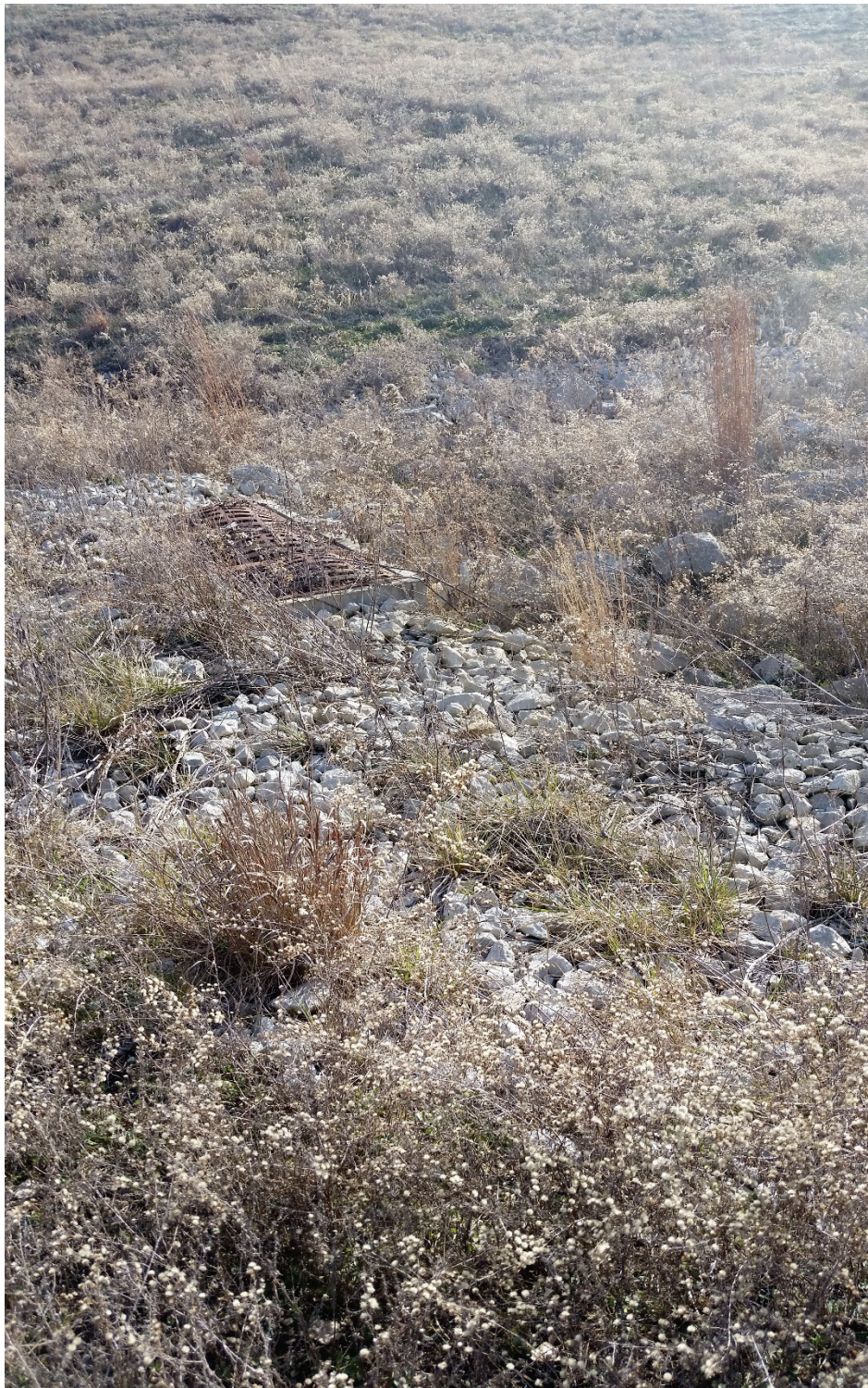
Photo 10: ES9 East Plant Area Cover
