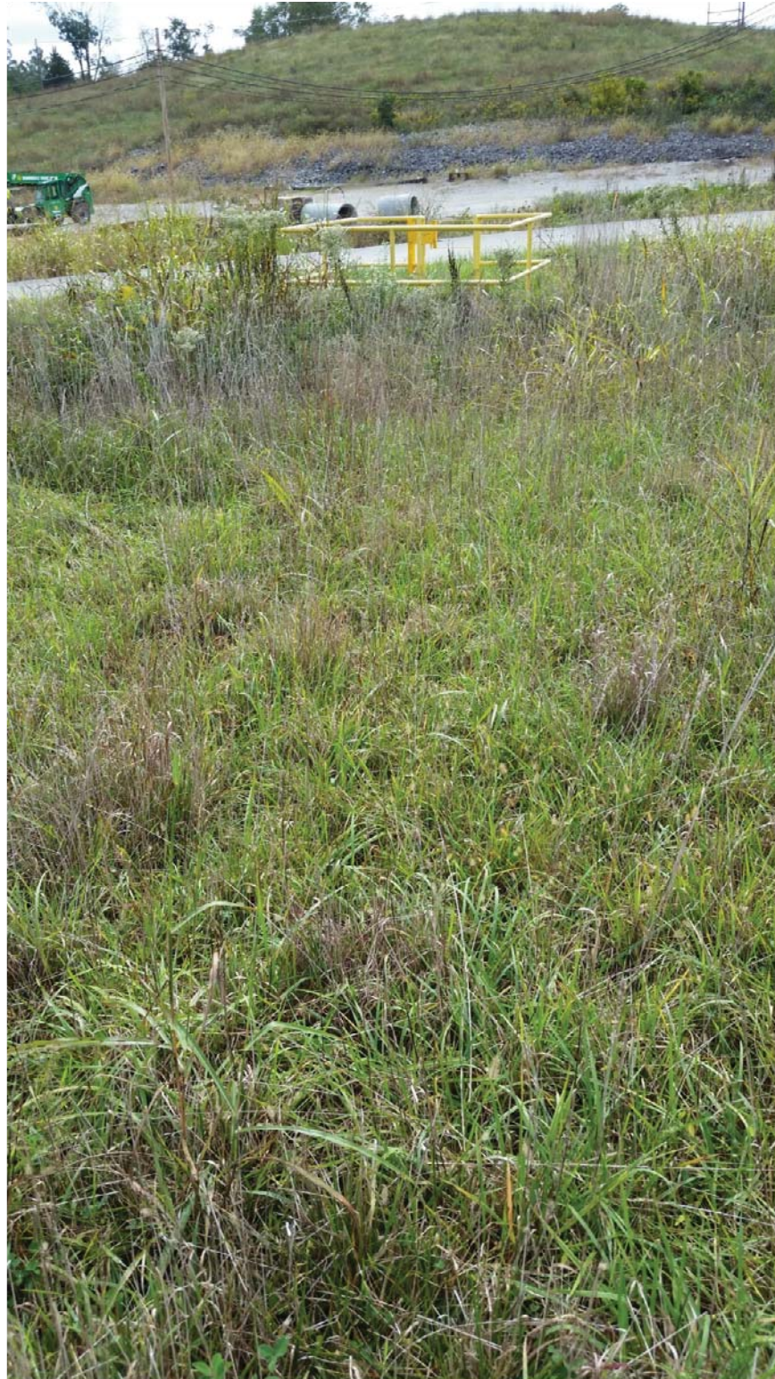
Photo 18: EV7 East Plant Area Cover facing south towards EV9.
