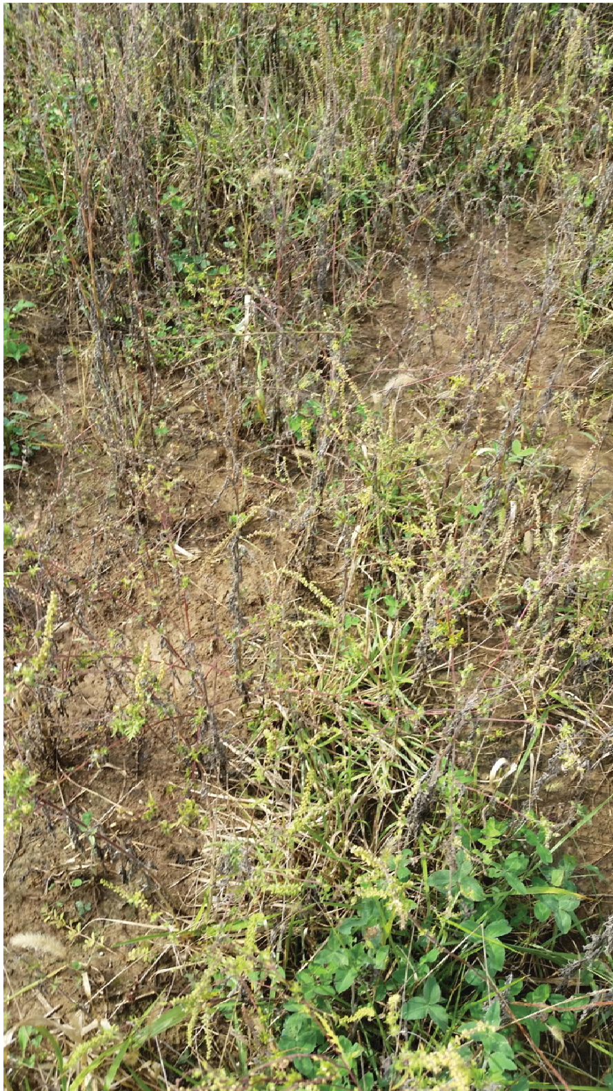
Photo 13: Slight topsoil erosion at ES12 East Plant Area Cover System.
