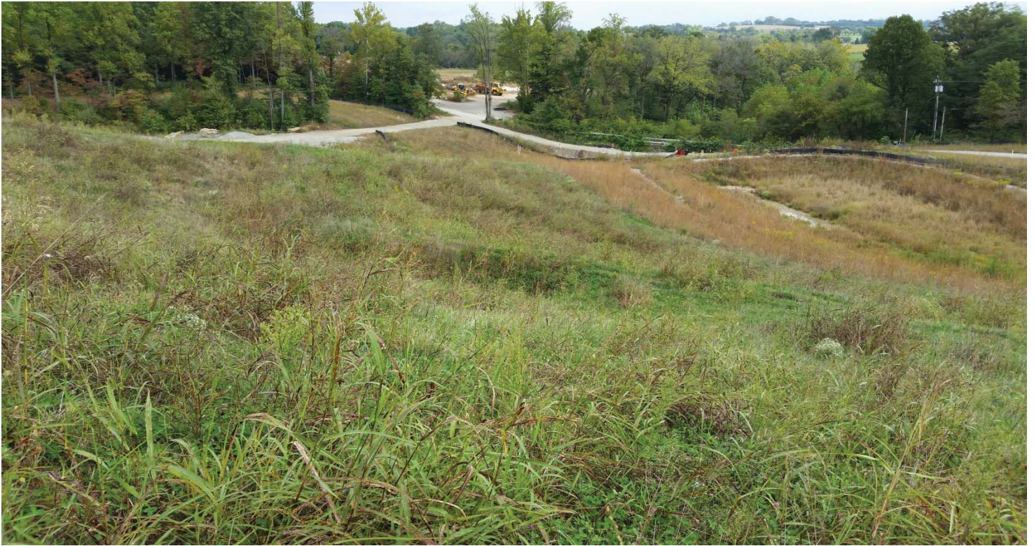
Photo 9: EV4 East Plant Area Cover looking northeast toward ES11 East Plant Area Cover.
