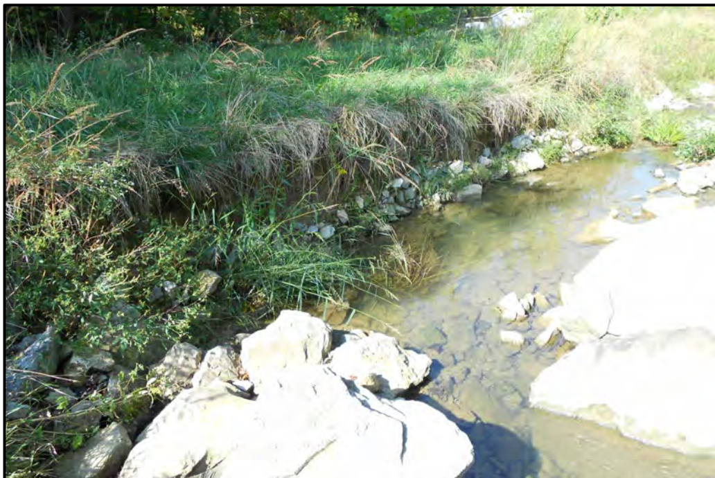
PHOTO 6: LOCATION 3 - LOOKING WEST (SOUTH BANK)
