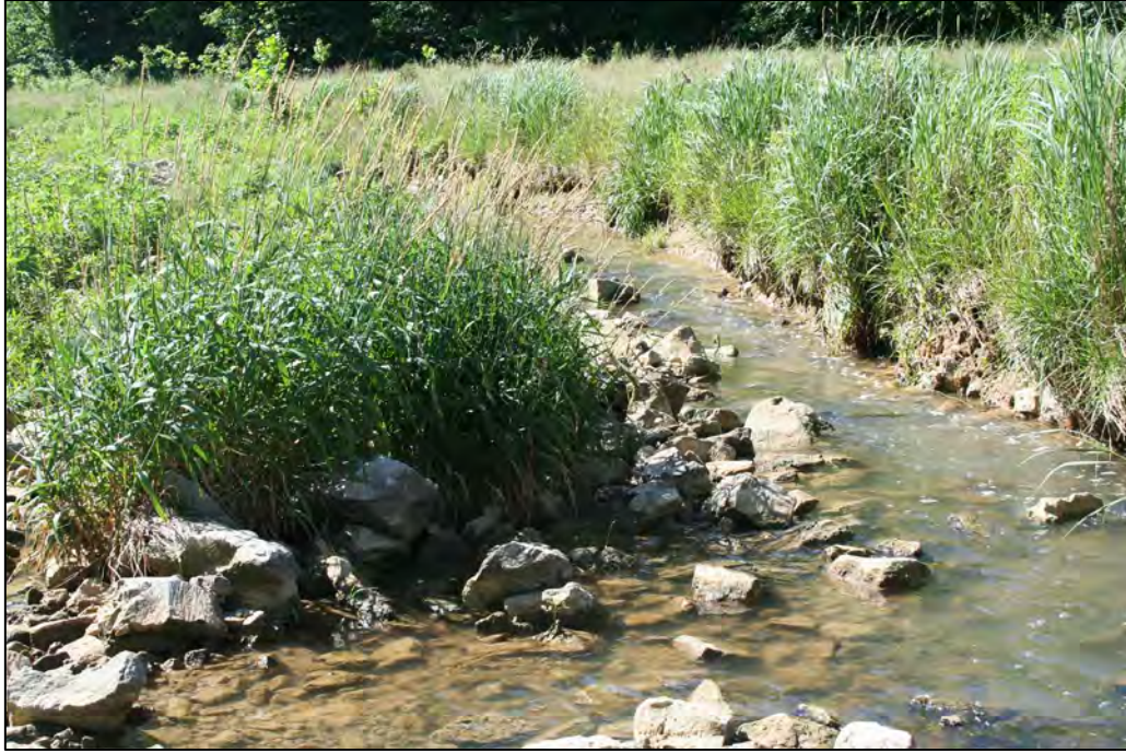
PHOTO 11: LOCATION 6 - LOOKING SOUTHEAST (UPSTREAM)
