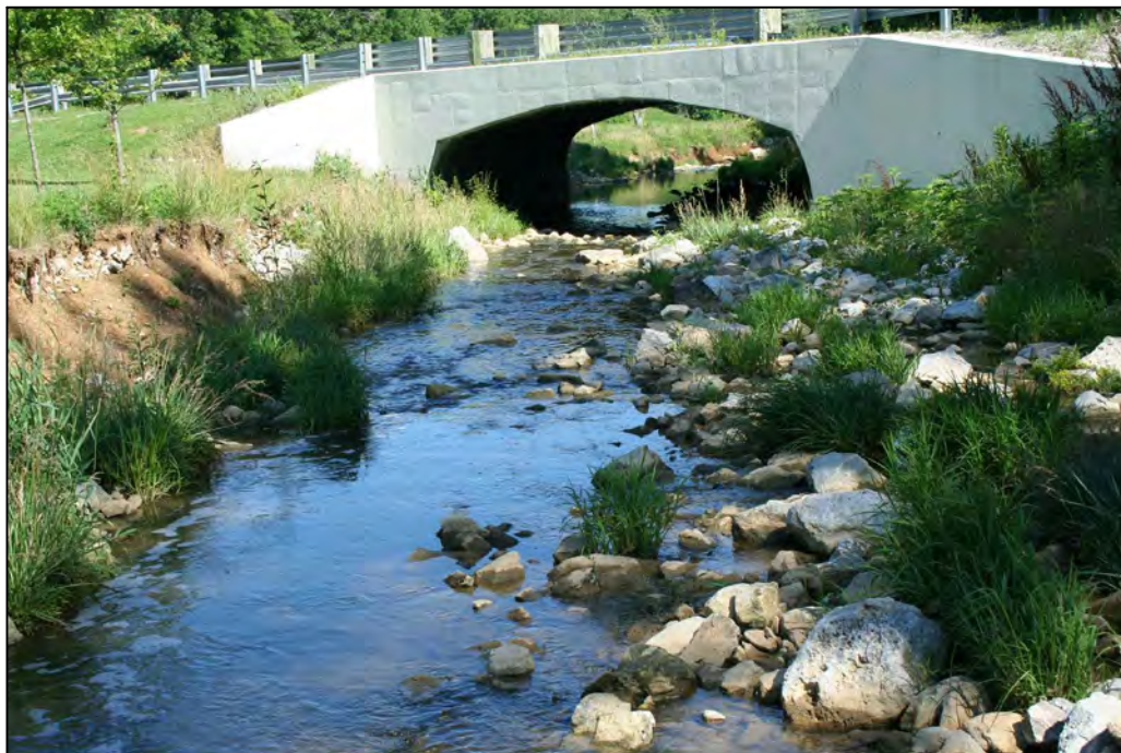
PHOTO 15: LOCATION 7 - LOOKING NORTHWEST
