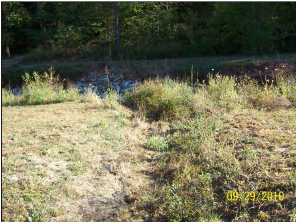
FIGURE 3.1 - PARCEL 22, LOCATION 3, DRAINAGE SWALE, LOOKING NORTH-EAST (DOWNSTREAM)
