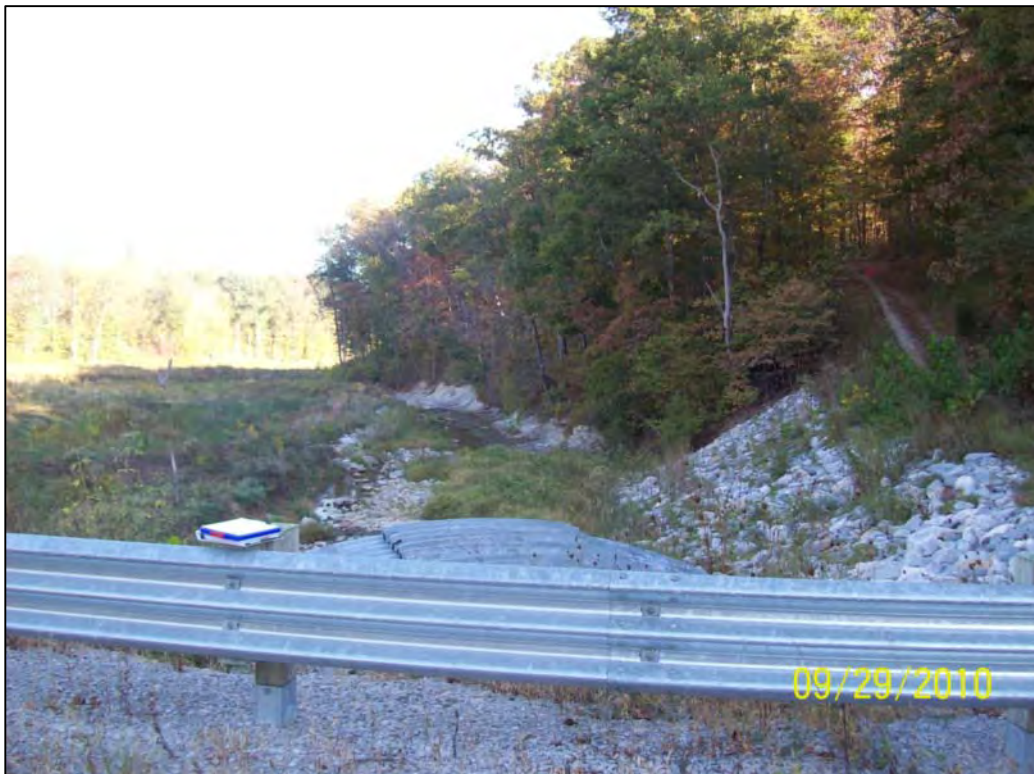
FIGURE 1.1 - PARCEL 22, LOCATION 1, LOOKING DOWNSTREAM
