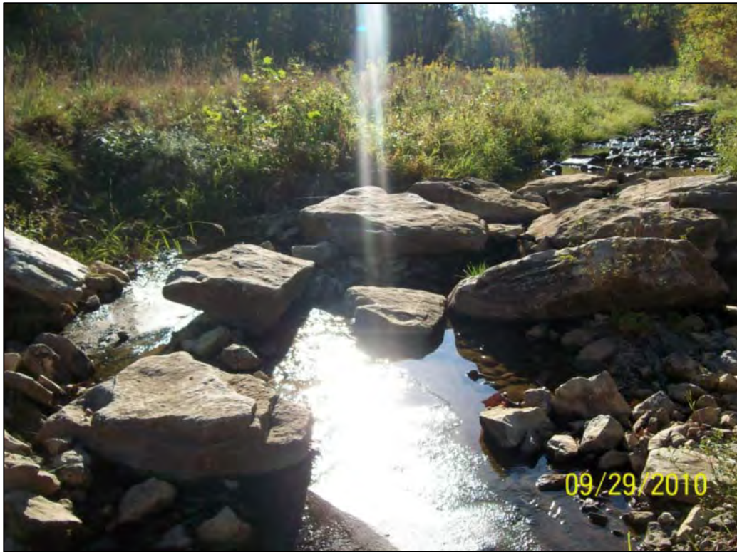
FIGURE 7.0 - PARCEL 22, LOCATION 7, FORCEMAIN CROSSING, LOOKING UPSTREAM
