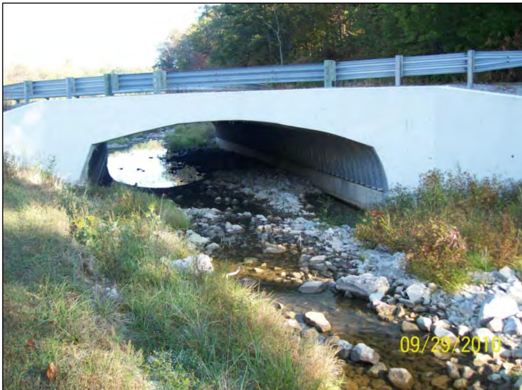
FIGURE 2.1 - PARCEL 22, LOCATION 2, LOOKING DOWNSTREAM
